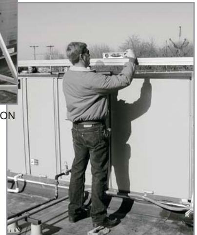
LEVELING THE COMPONENTS
