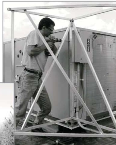
CORNER TRUSS INSTALLATION
